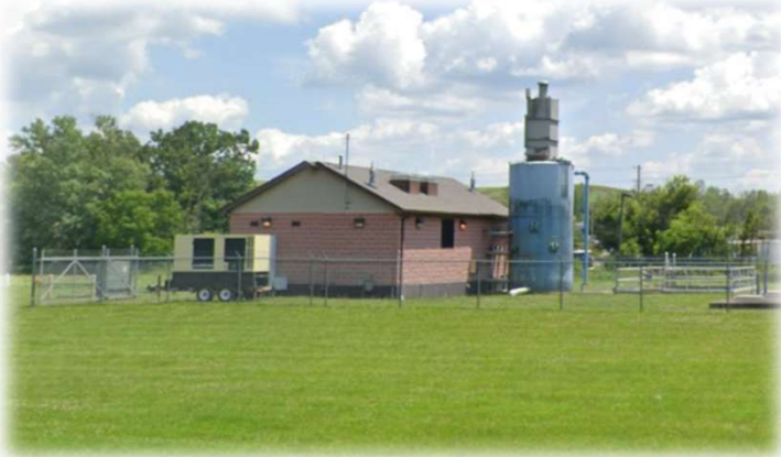
Baltic Water Treatment Plant
